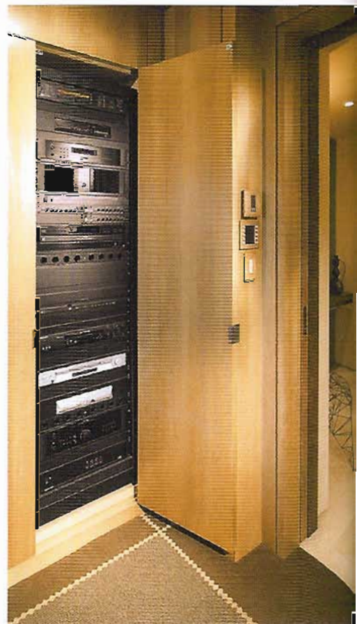
Two disparate lighting controllers—one a professional museum-style fiber-optic system, the other a traditional residential Lutron HomeWorks system—had to be integrated seamlessly via the Crestron touchpanels.
