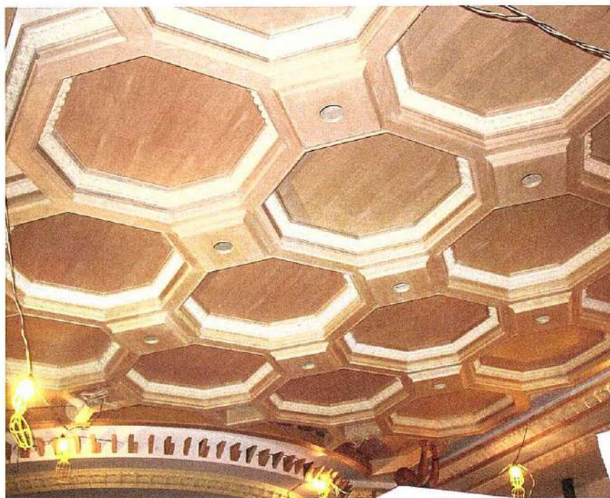
An intricate coffered ceiling design in the upscale home theater installation took away about 9in. of height, requiring reframing of the raked risers on which the theater seats would be placed.
